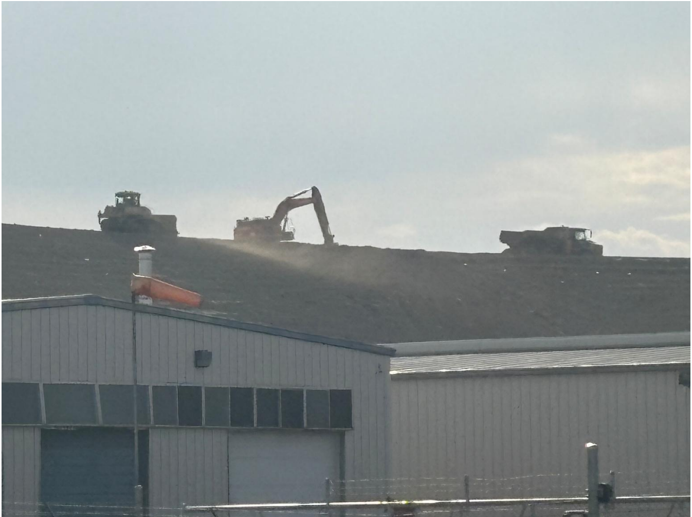
Clean Harbors capping activities, September 29
